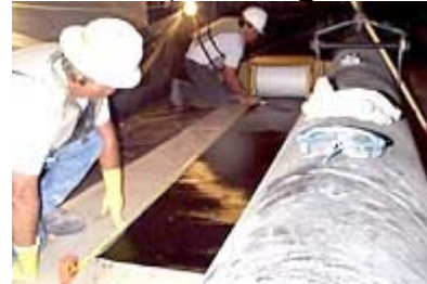
Photo: 5 (Patching with Repair Mortar)
