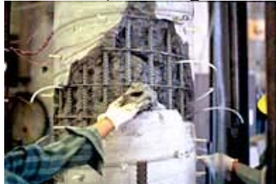
Photo: 4 (Patching with Repair Mortar)
